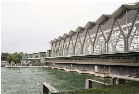
17 Kraftwerk Birsfelden, Switzerland, 1951, Hans Hofmann
