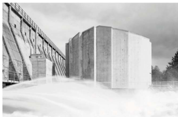
26 Pálsbu Hydro Power Station, Tunhovd, Norway, 2007, Manthey Kula Architects
