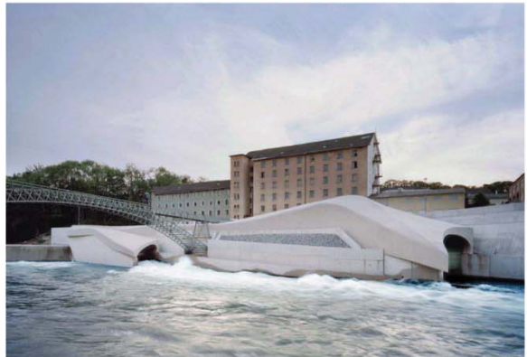
25 Hydroelectric Power Station Kempton, Germany, 2010
